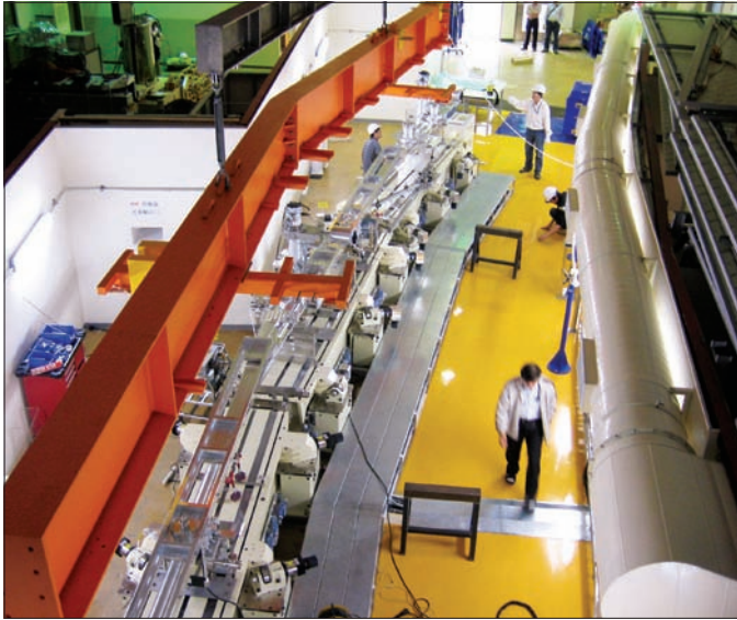
A 14-m long "hanger", equivalent in size to the vacuum chamber, was built to carry the assembled unit.
