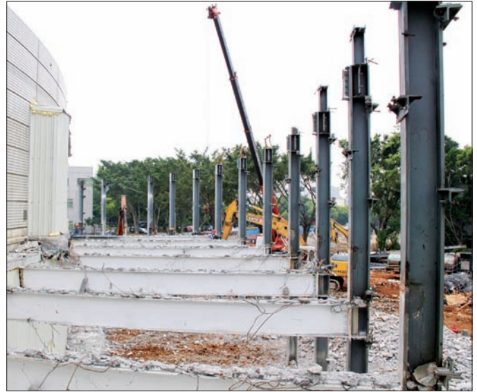
Walls of the TLS building were torn down for the new interface with the TPS storage ring and piles were inserted to stabilize the TLS foundations.
